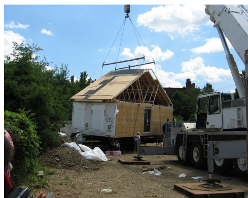
Second floor module lifted from truck bed
