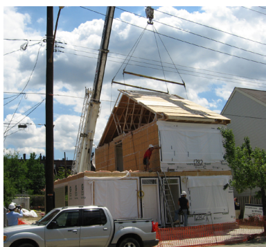
Second floor module being craned into place
