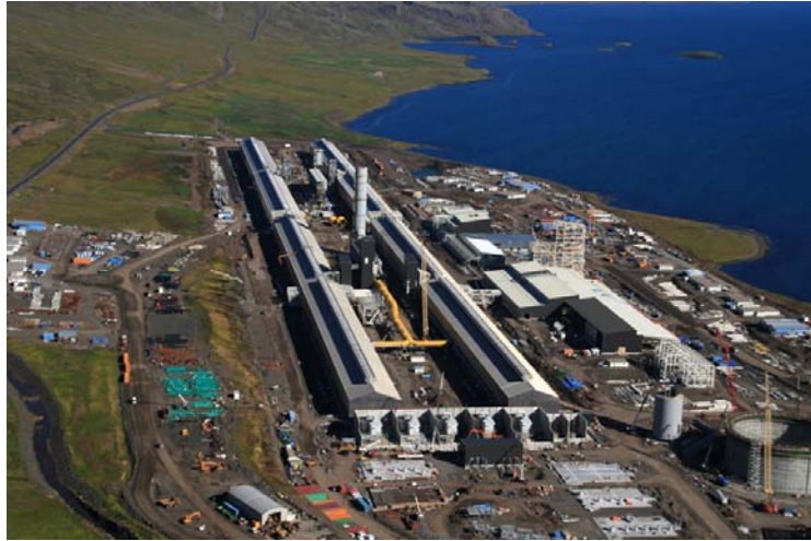
Smelter under construction
