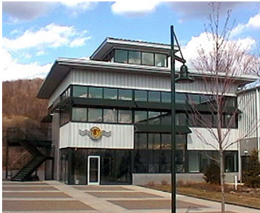
restaurant structure is part of sports complex
