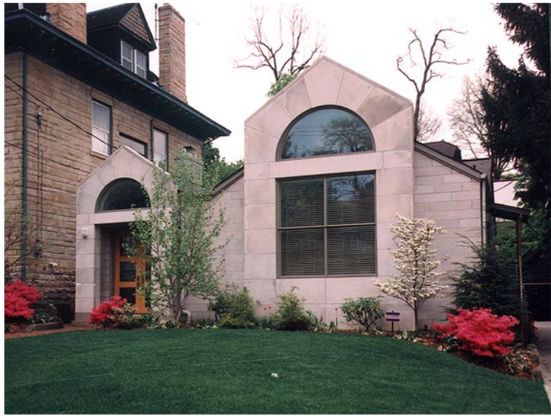
Portion of front facade was extended and finished with lime stone
