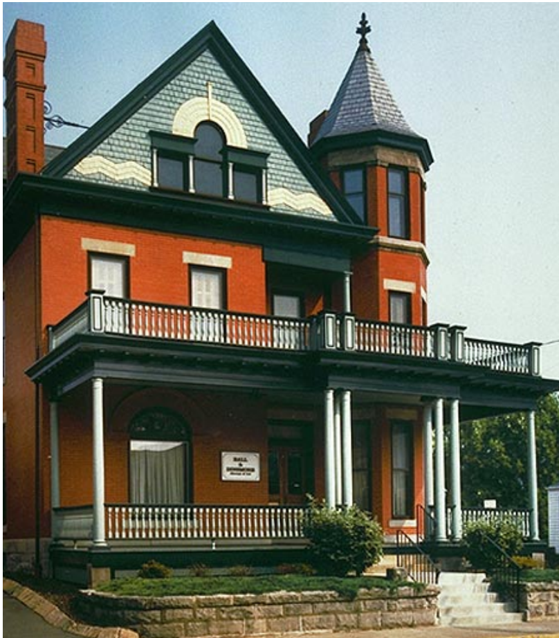
After the renovation
