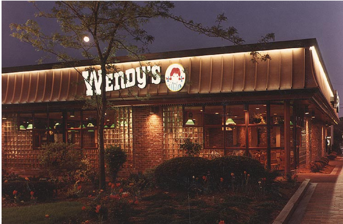
exterior addition renovation to original prototype store
